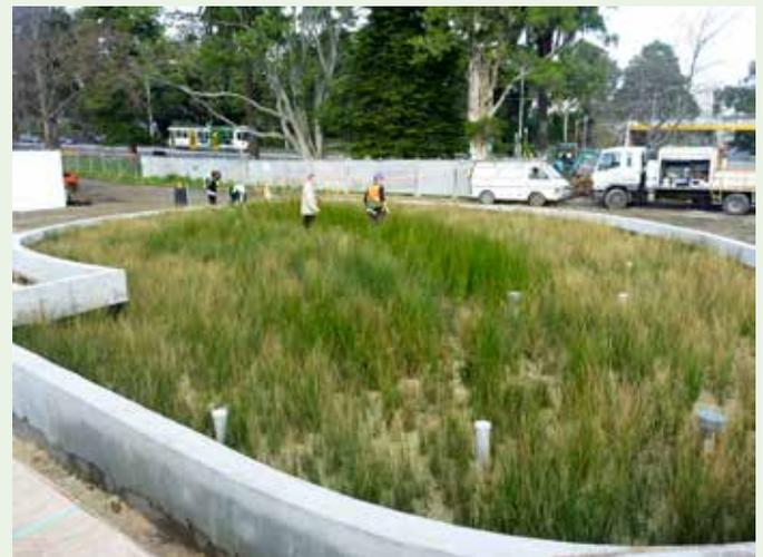
↑ The 240m<sup>2</sup> biofiltration bed used at Fitzroy Gardens has a footprint that's just 10% of a standard gravity-feed system. A slightly coarser sand was used to handle the regular pumped inundation of the bed; this also affected plant selection of *Juncus procerus* and *Juncus gregiflorus*.
