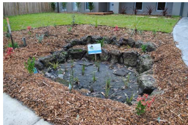
Figure 1. An example of the stormwater infiltration systems installed as part of the Little Stringybark Creek project.
