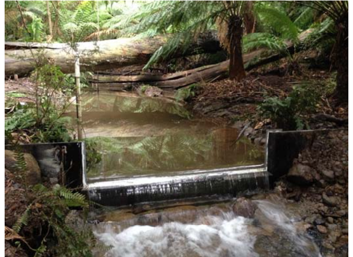
Figure 2. An example of the weirs used to measure the creek’s hydrology (reference stream).
