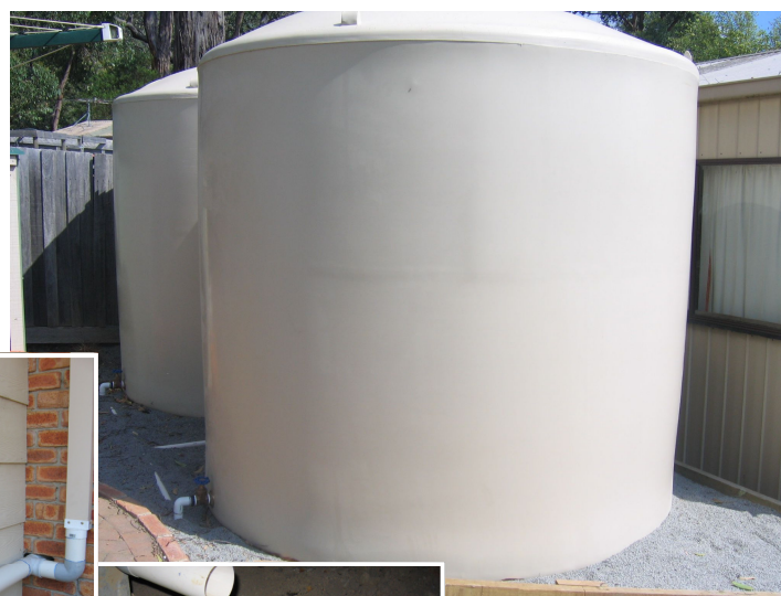
Two down pipes are joined (far left) in order to redirect them into a collection pit (left) from where the stormwater from all the roof is pumped into two 9,000 litre tanks (above).
