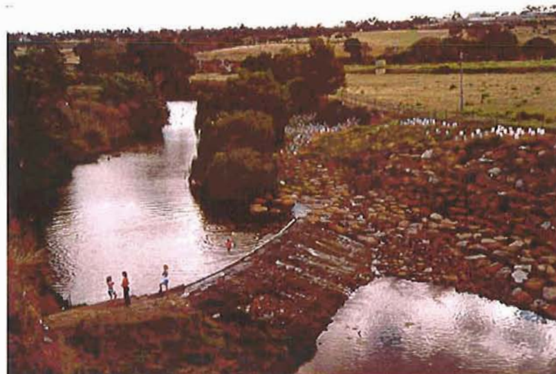
Figure 8. Arundel Street weir looking upstream (chainage 12 km), with recently installed fishway on left bank.
